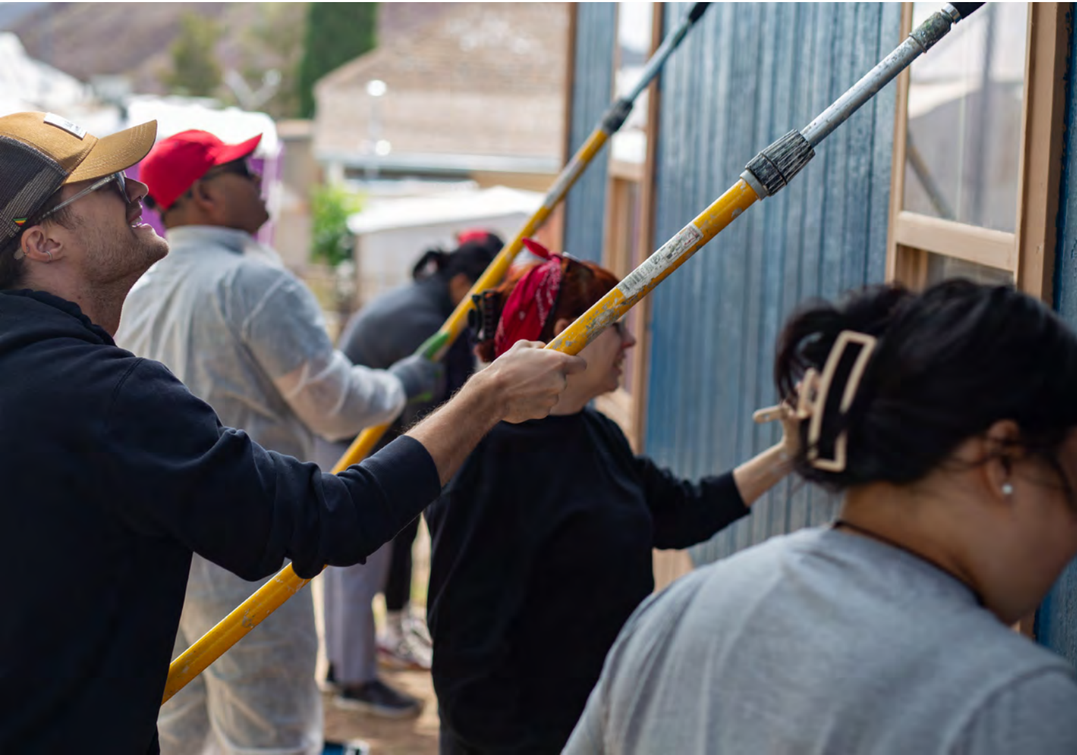
RHPP Service Learning students, Cameron Dockens and Shunrang Chin working on home repairs with Step Up Bisbee/Naco
